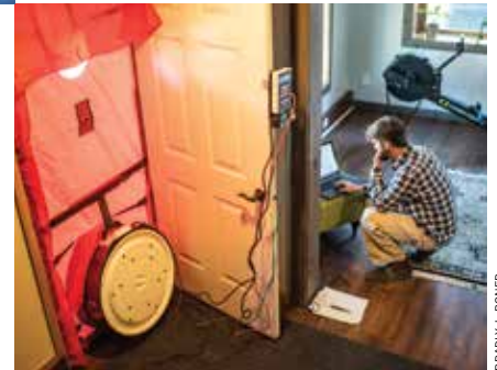
Paulson's process during an energy audit involves sealing up a building and using a blower door to find air leaks.
