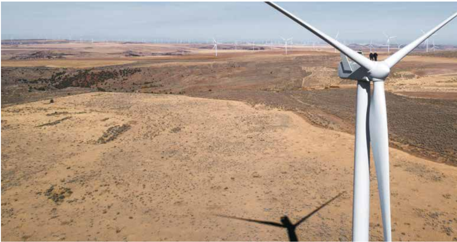
The Horse Butte Wind Farm southeast of Idaho Falls, Idaho, provides green energy to Lower Valley Energy customers.
